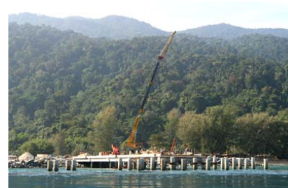
Tekek Marina in construction
